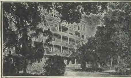
Part of Main Building
