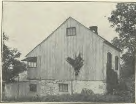
Fig. 4. Defective building in the country—great absence of window space. Five deaths from tuberculosis since 1896.
