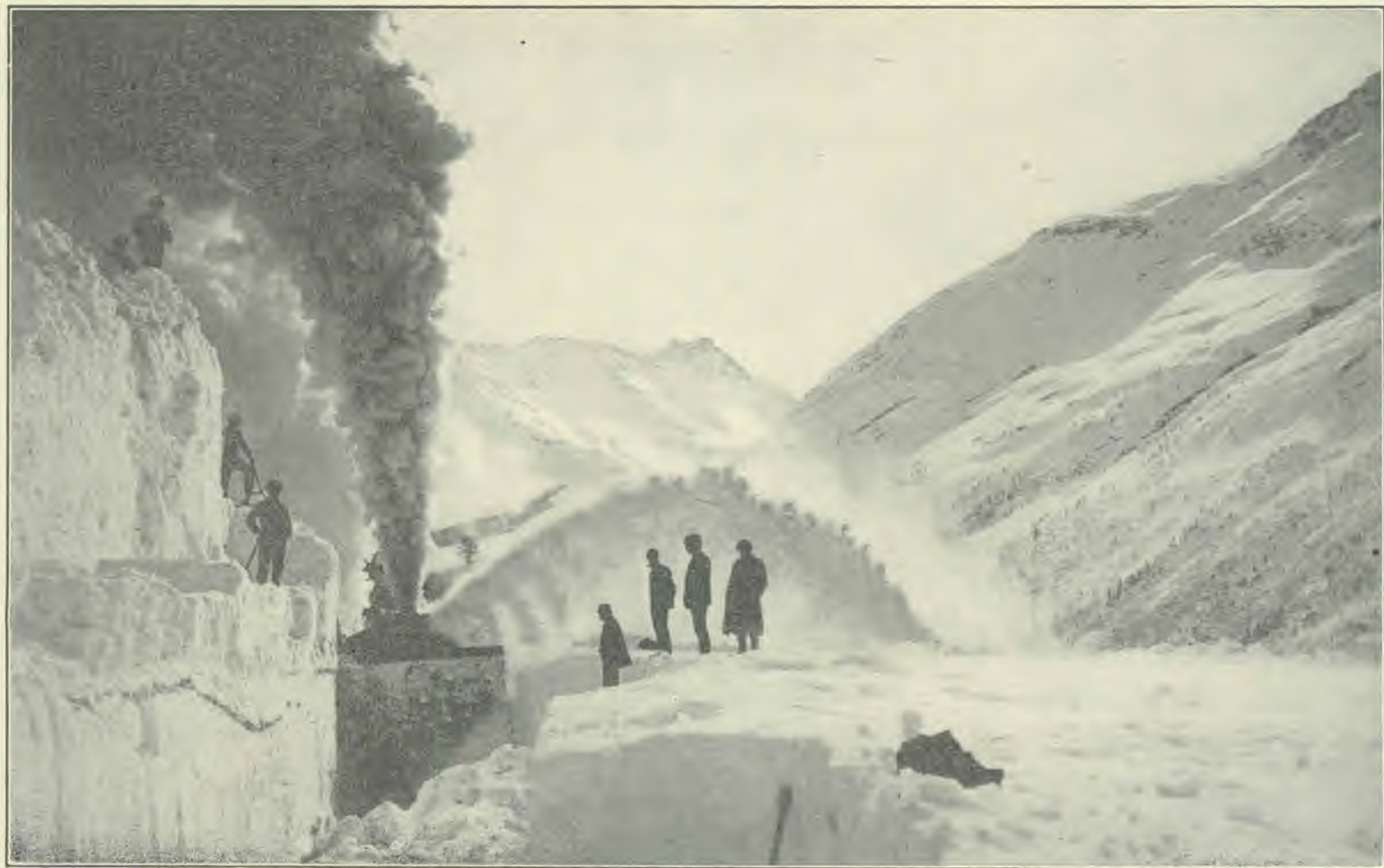
ROTARY PLOWS CLEARING THE TRACK IN A MOUNTAIN PASS
