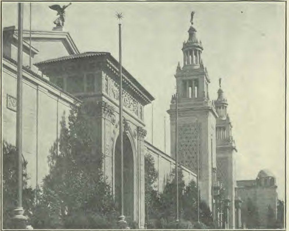
DOORWAY, PALACE OF LIBERAL ARTS, SHOWING TOWERS
