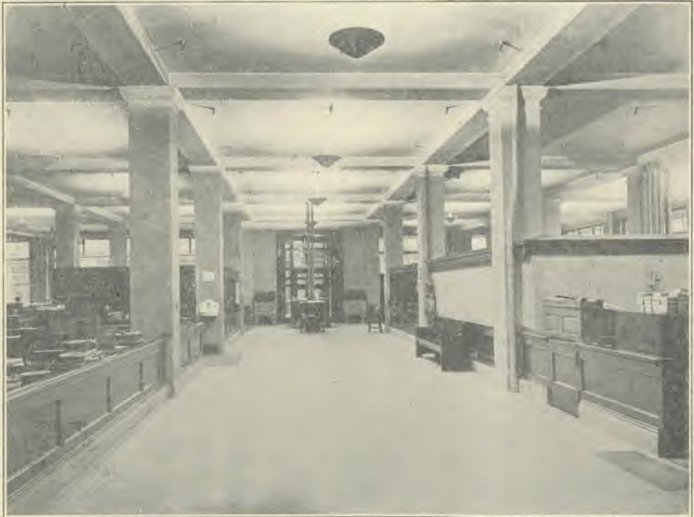
Courtesy General Electric Company
