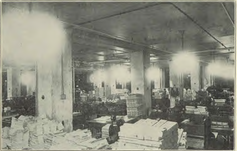
Courtesy General Electric Company
