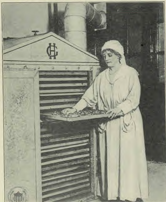
Mrs. Oliver Harriman, of New York, working a dehydrating, or food drying, machine. Mrs. Harriman has established a food research laboratory to further the preservation of food.
