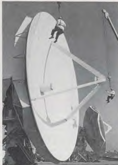
Space Trapeze—Engineers take to old-fashioned bosun's chairs to make adjustments on the forty-foot antenna that constitutes one ground-link terminal in the United States Army's satellite communications system. The air-transportable antenna, largest of this kind, can be taken apart and erected along the line of a child's erector set, as the rear view of the second antenna shows.
