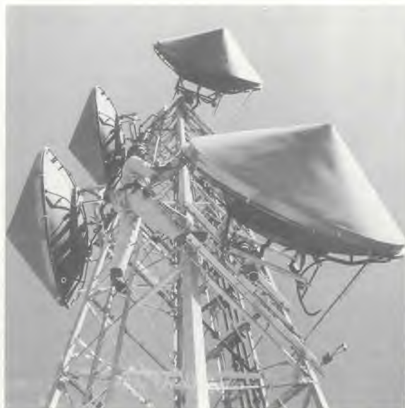
These disk-shaped reflectors send and receive narrow beams of radio waves as part of an expanding communications network linking points on the Union Pacific Railroad.
