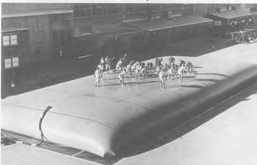
Snapping into a running play atop 210,000 gallons of water, the Agua Fria High School football team of Avondale, Arizona, is perched on one of the world's largest flexible storage tanks. The collapsible tank was made for the Army for use in storing fuel in combat areas.
