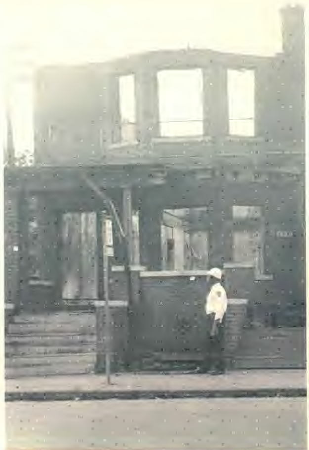
Elder C. B. Rock, pastor of the City Temple Church in Detroit, is shown examining one of the buildings gutted by fire during the riot.
