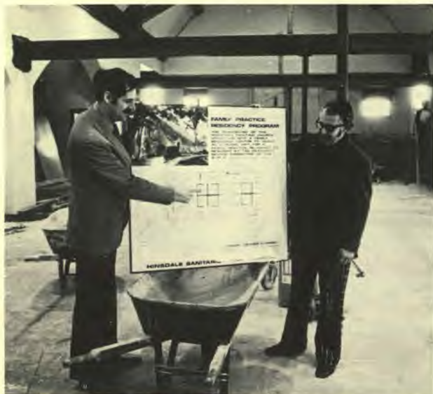
Construction is going on in Oak Hall as the building is readied for occupancy by the Hinsdale Family Medicine Center this spring. Drs. W. Duane Dodd, left, and Everet W. Witzel, directors of the center, examine plans for the structure.
