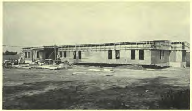
New office under construction
