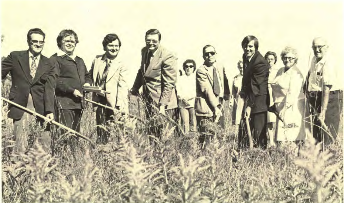
Members of the Sturgeon Bay Church broke ground August 17 for a new edifice. From left are Don Mann, elder and chairman of the building committee; architect George "Pat" Mangan; associate pastor Steve Shipowick; conference president Robert L. Dale; Floyd Knuth, building committee member; Pastor Andrew Mustard; Lorriane Nelson of the building committee, and Cedric Mann.
