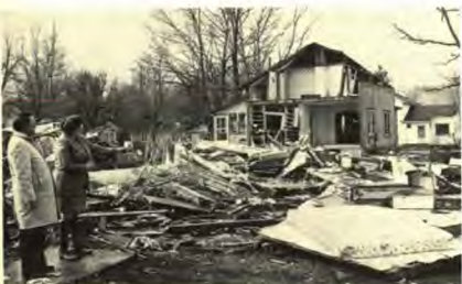
Elder Buckman and Mrs. Renshaw examine the ruins of one home hit by the tornado in Augusta.
