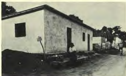
SAWS recreated these neat cement block homes. More than 1,000 are now finished throughout Guatemala.
