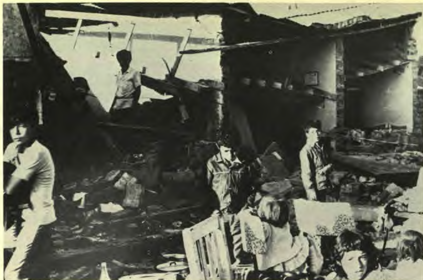
Guatemalan homes were in shambles after the earthquakes.
