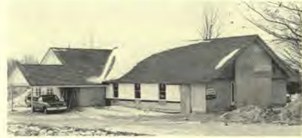
Partially completed new Sturgeon Bay Church.
