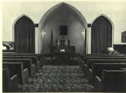
Remodeled Menominee Church
