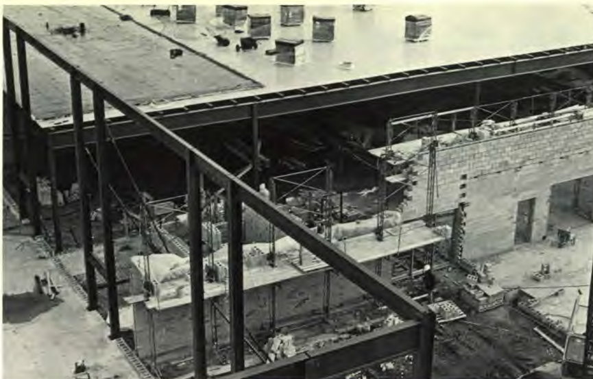
Construction is well underway at Andrews Academy.
