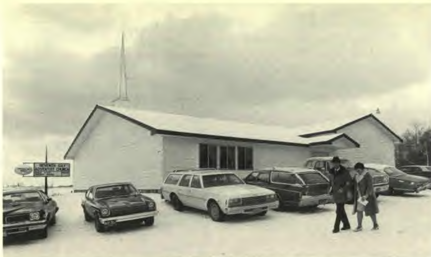
This is an exterior view of the West Branch Church which was constructed from two portable classroom units.
