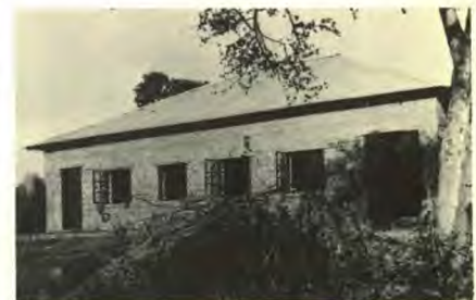
This one-room building at Bangladesh Seminary is divided into four classrooms by burlap partitions.
