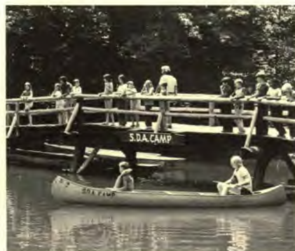
The bridge across Little Grassy Lake is being rebuilt this winter to provide better access to Vesper Point and waterfront activities such as canoeing.
