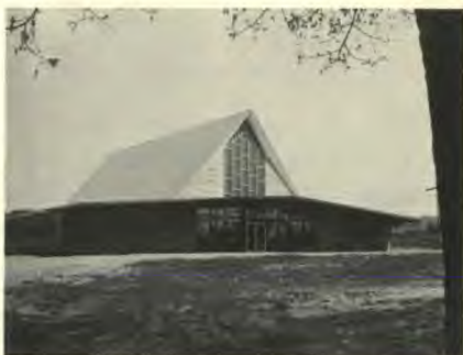
The new Decatur-Glenwood Church
