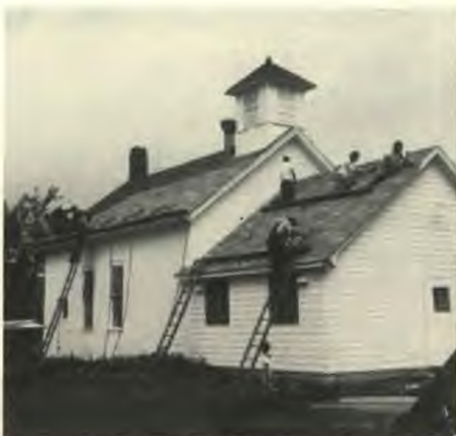
. . . and during renovation.
