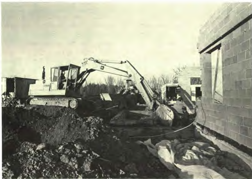
When construction of the new home of Chippewa Valley Hospital and nursing Home, Durand, Wisconsin, is completed, the facility will have 30 hospital beds and 60 nursing home beds.
