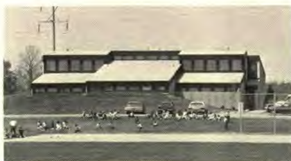
The Holland School is designed for fuel efficiency and energy conservation.
