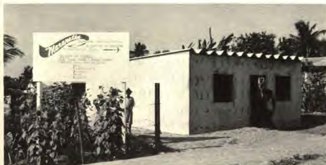
Above: Purchasing and transporting heavy equipment was a major task to be accomplished before the disaster relief project could begin. Left: The 160 homes built were poured concrete structures.
