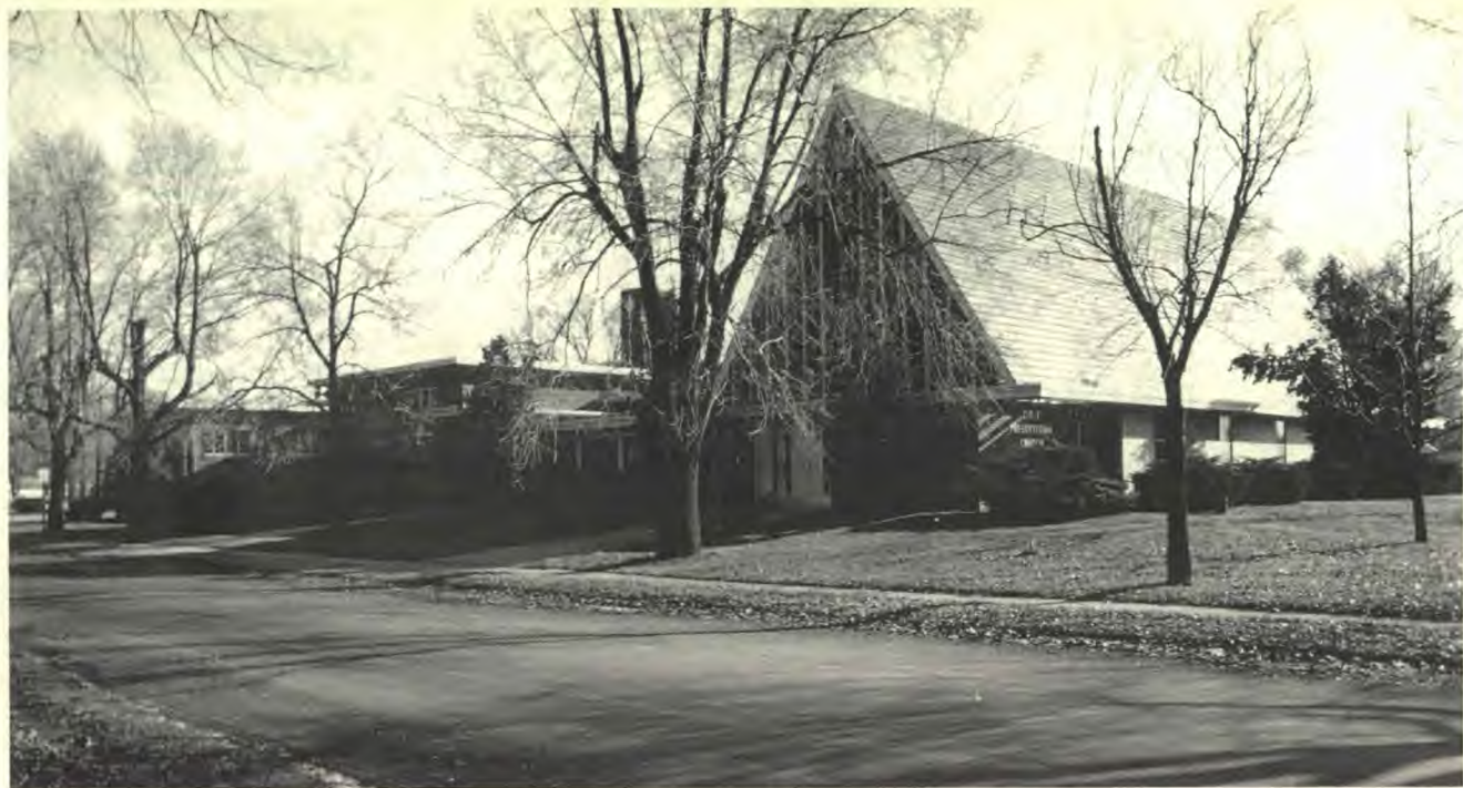
The new Reid Memorial Church in East St. Louis.
