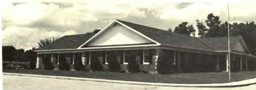
The Indiana Conference office is located along Highway 31, one mile north of Carmel, Indiana. The office was moved from Indianapolis in the fall of 1975. Its rural setting now provides a peaceful atmosphere for workers.
