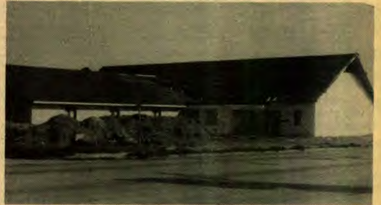
The new Racine church building is being constructed.
