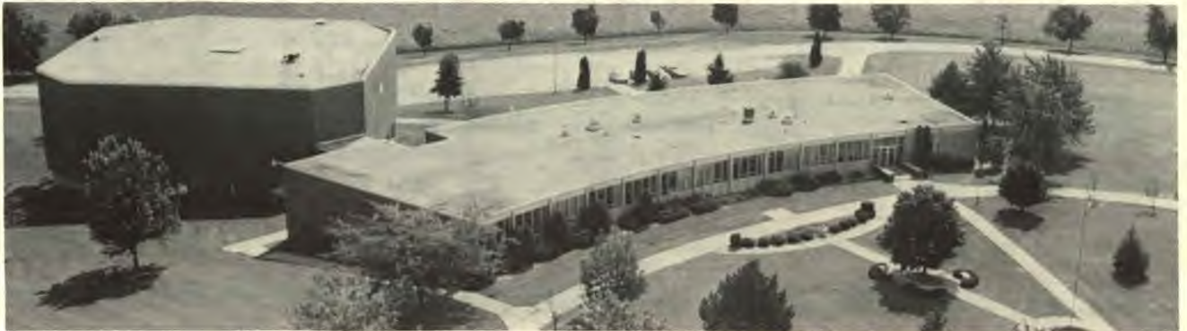
Broadview Academy Administration Building and Music/Chapel Building
