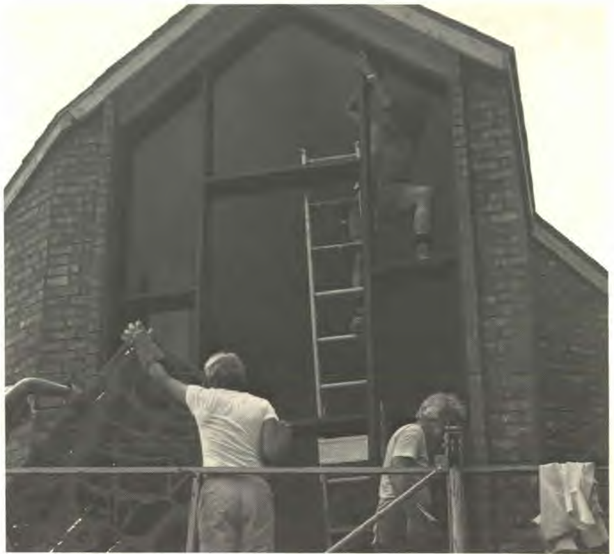
Workers install one of the stained-glass windows.
