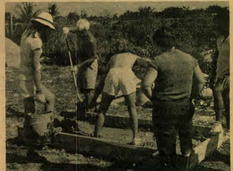
Mixing cement by hand at the New Providence Church
