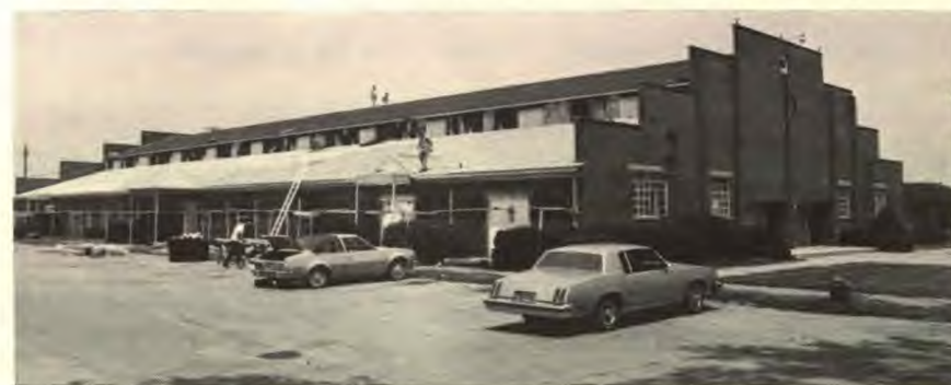
The remodeling of the gymnasium includes a new roof.
