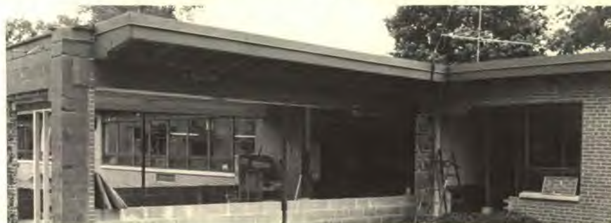
Extensive renovations are taking place in the administration building.
