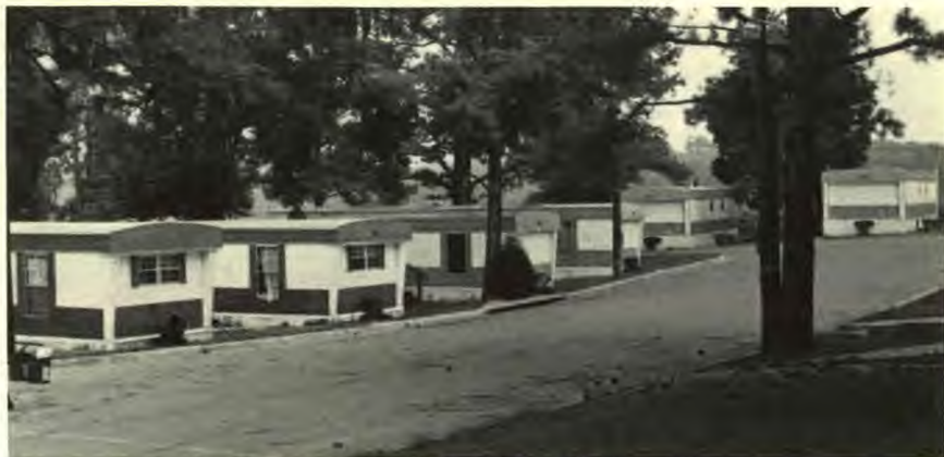
When the enrollment doubled at Oakwood College last year, many of the students found their assigned "dorm rooms" to be in house trailers. Adventists in the Lake Union will have an opportunity to help Oakwood College cope with this enormous growth by giving to the Oakwood College Annual Offering on August 10.
