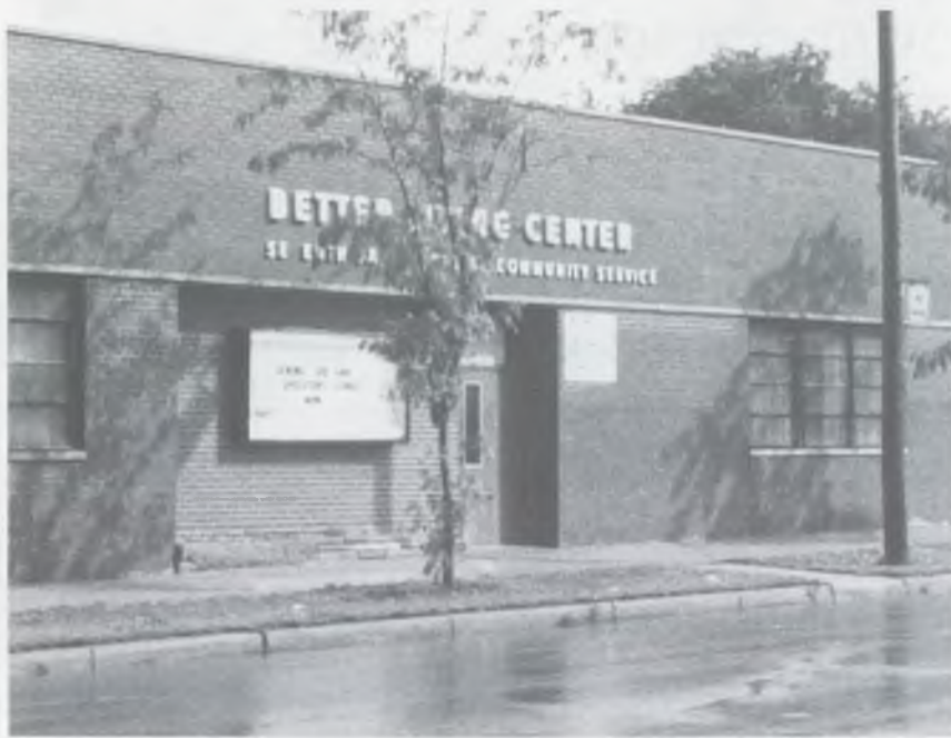
The Detroit, Michigan, Better Living Center, located at 3240 Puritan Street, is one of three centers operated within the Lake Union Conference. Don A. Copsey, inner-city coordinator, says there are plans to open a fourth center in Indianapolis, Indiana.
