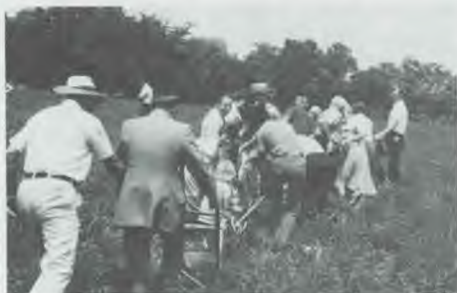
Elder Archie Moore guides the plow as Cicero Church members pull to break ground for the church.
