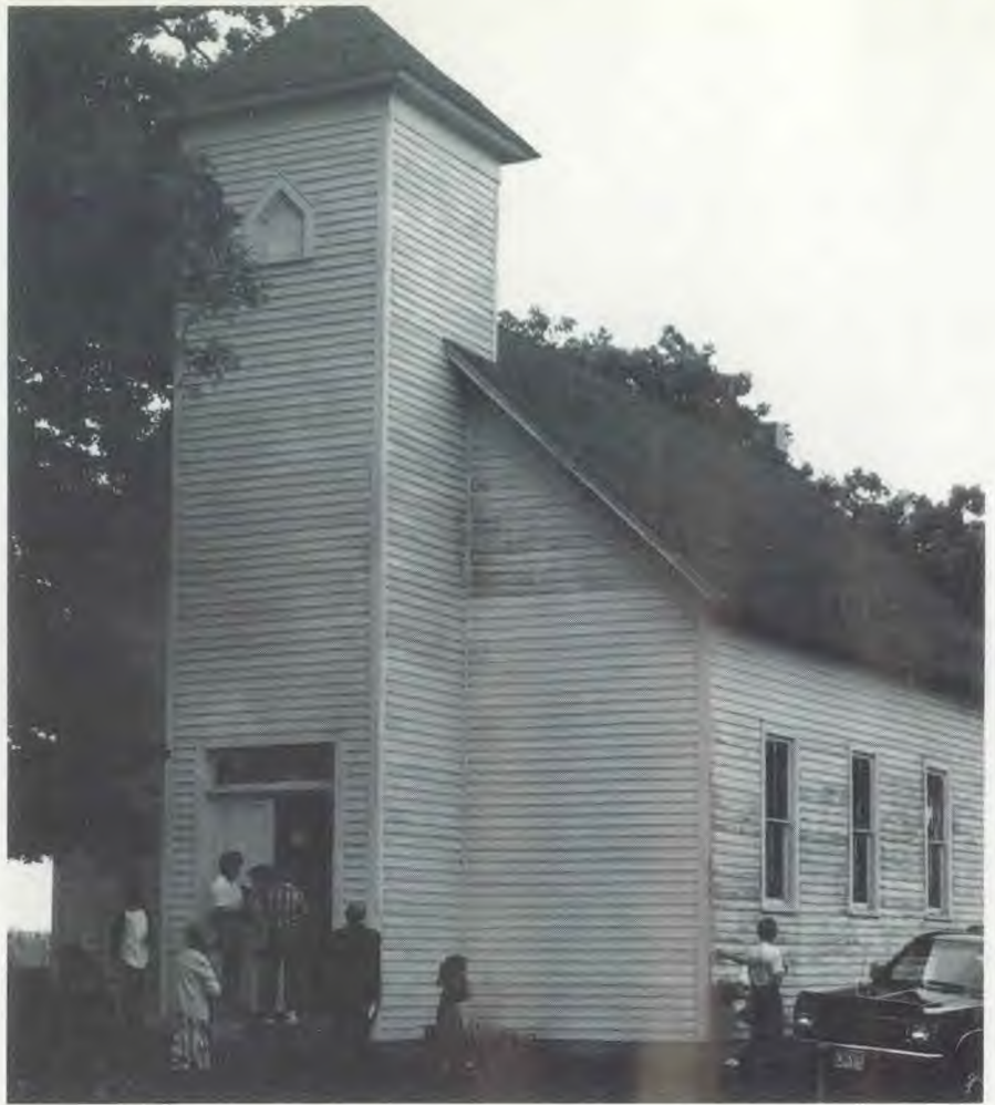
The Waterloo, Wisconsin, Church built in 1912 is used once a month for Sabbath afternoon services.
