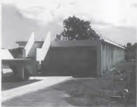
Arriving project volunteers found the building ready for the second story.
