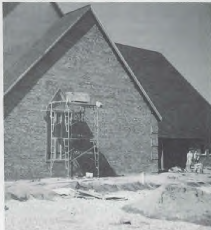
Maureen and LaRae Plumb stand in front of the almost-completed Greenwood Fellowship Church-Elementary School complex.
