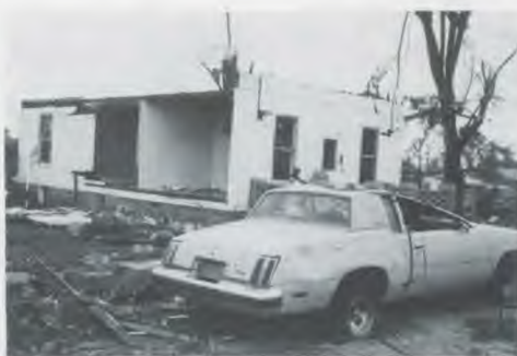
Scenes of destruction in Petersburg, Indiana, after the June 2 tornado.
