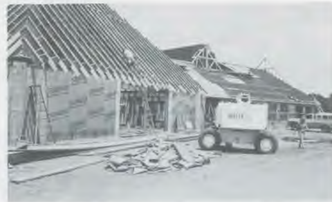
The Korean Seventh-day Adventist Church in Berrien Springs, Michigan, under construction.
