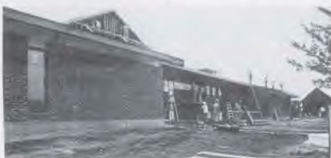
The Aurora Educational Center nearing completion.
