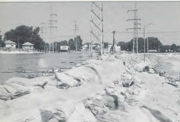
A flooded portion of the river in south St. Louis, MO, pushes against the weakened levee.
