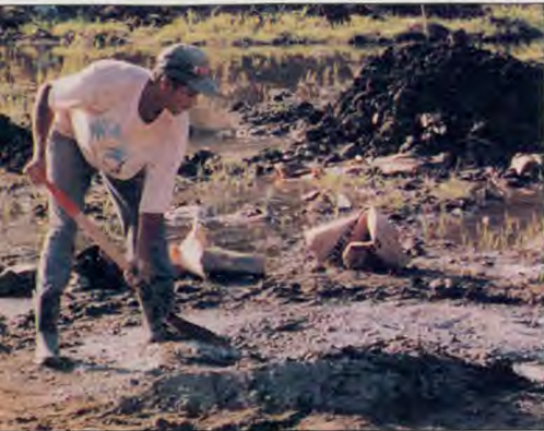
To keep up with workers demands, mortar was mixed on the ground.
