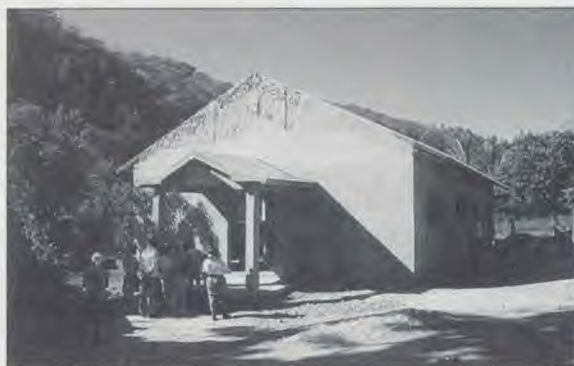
In the very poor village of El Coco there are 125 SDA members. For seven or eight years this congregation had only a foundation for their church building. Now the church is a structure (pictured above) as the result of $6,000 given to them by the Michigan Conference. However, it will take another $5,000-$6,000 to complete the church's interior.
