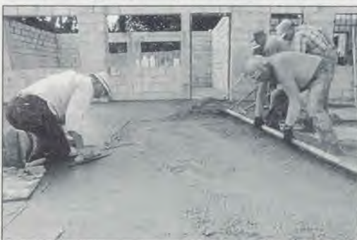
Andy Snyder (right, front) led out in laying the 7,040 square feet of floor for a six-room school in Escuintla, Guatemala.
