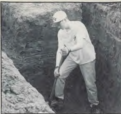
Alan Gatward digging for the septic system. (Photo by Jim Gatward.)
