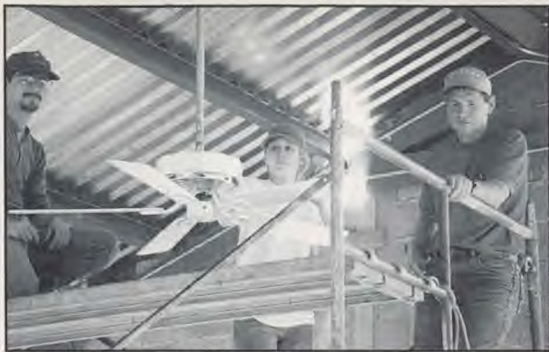
From left: John Reinbold, Kelly Payne, and Steve Vail, electrical crew members. (Photo by Alan Gatward.)
