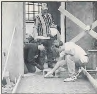
John Johnson checks out the progress of the sidewalk by Mike Dixon (left) and his son Mike. (Photo by Alan Gatward.)
