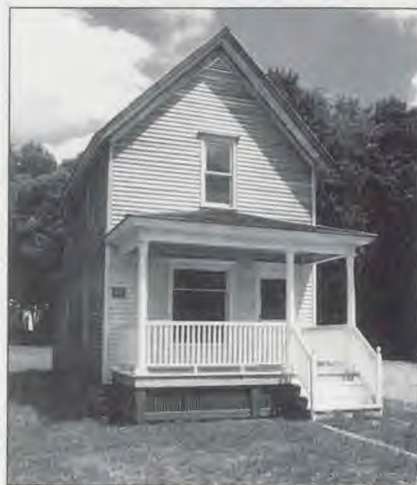
Restoration of the exterior of the J. N. Loughborough house is nearly complete, but the interior awaits restoration.
