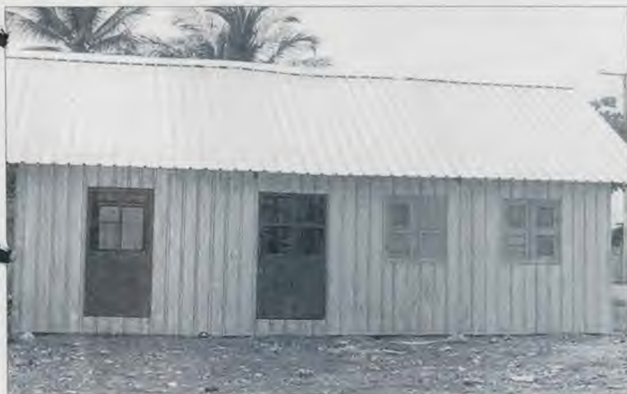
The portable chapels of the East Dominican Mission are made of steel and are bolted together so that they can be taken apart and moved to a new location. The members of the Illinois Conference donated the money for five of these structures.
