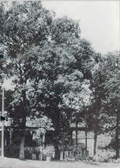
An early photo of Hinsdale Hospital
