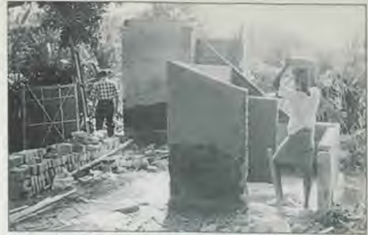
The funds sent also helped with construction of new latrines.
