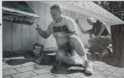
From left: Keith DeBarr and Joe Whitaker, Charlotte Church members, work on painting the second story of the food bank.
