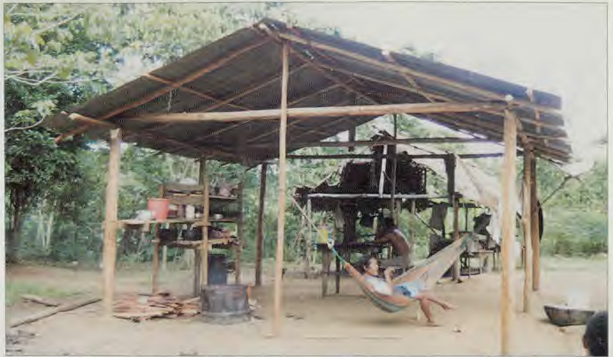
Jungle houses are designed for maximum cross-ventilation.
