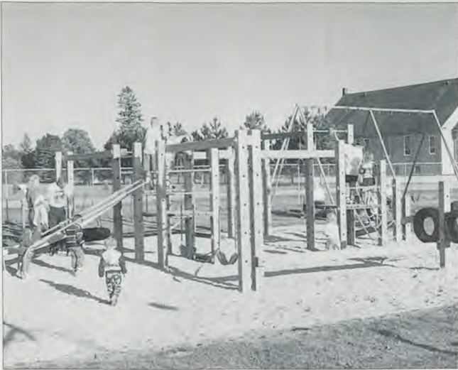
New playground equipment is installed at Wilson Junior Academy.
