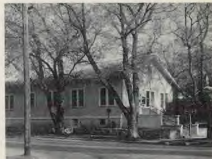
The first Casper Church, located at the corner of South Oak and West 12th Streets. Built in 1924, dedicated October 31, 1925, cost $9,000.00
