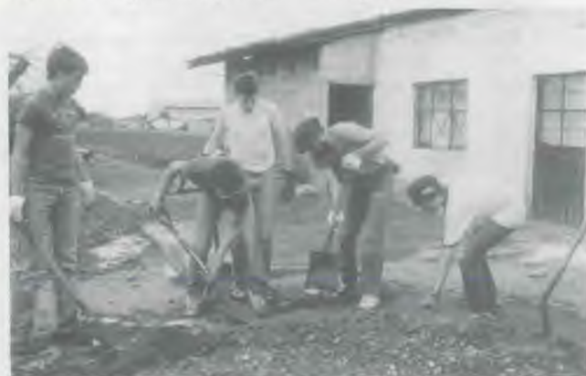
Chuck Hagele, Darin Horst, Shannon Nelson, Tim Simon, CVA religion instructor and John Buxton are seen working on a large pile of concrete mix for the church floor.
