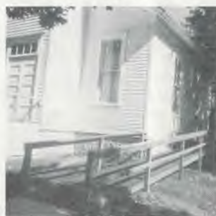
Grinnell church with new ramp.
