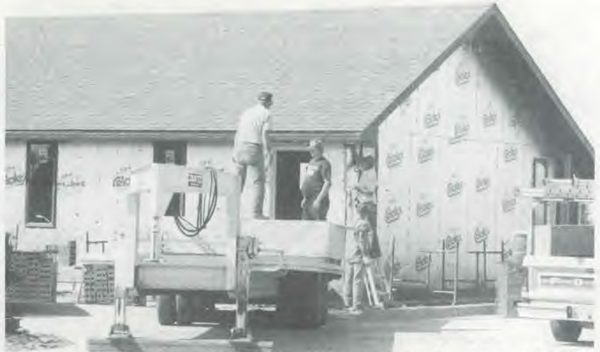
The new Goodland, Kansas church was raised in a little less than three weeks with the help of Maranatha Flights International volunteers.
